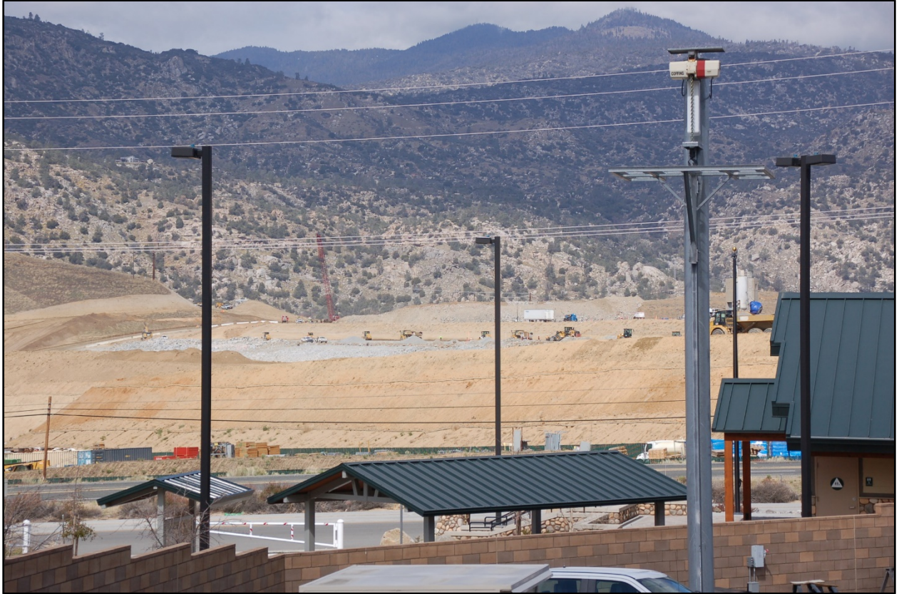
Figure A-4. Photo of the interim visitor center location. Fire station is shown on the left, while the Auxiliary Dam undergoing construction is in the background, along with views of the surrounding foothills.
